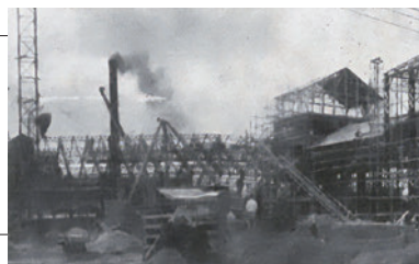
NPK compound fertilizer plant under construction
