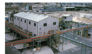
Multipurpose production facility for organic fluorine (1984)
