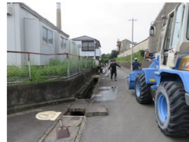
Road Gutter Cleanup Efforts in the Chikko District
