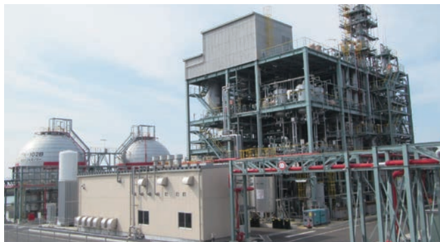
Our Ube UF-1 Plant, where HFO-1233zd(E) is manufactured
