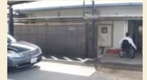
Example of barrier-free entrance (Matsusaka plant)
